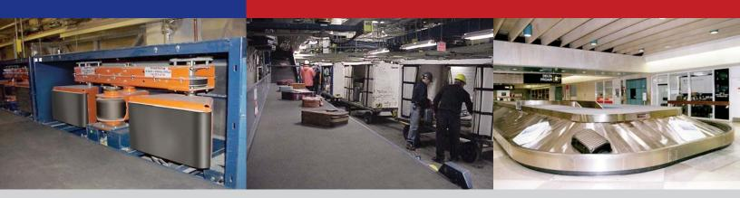
Horizontal sorting devices divert bags to adjacent make-up destinations as directed by the WebbView baggage handling control system. Inbound baggage is placed on belt conveyors that lead to the appropriate baggage carousels. Arrival passengers can pick up their baggage from a quiet, heavyduty sloped plate carousel (or a flat plate carousel).
